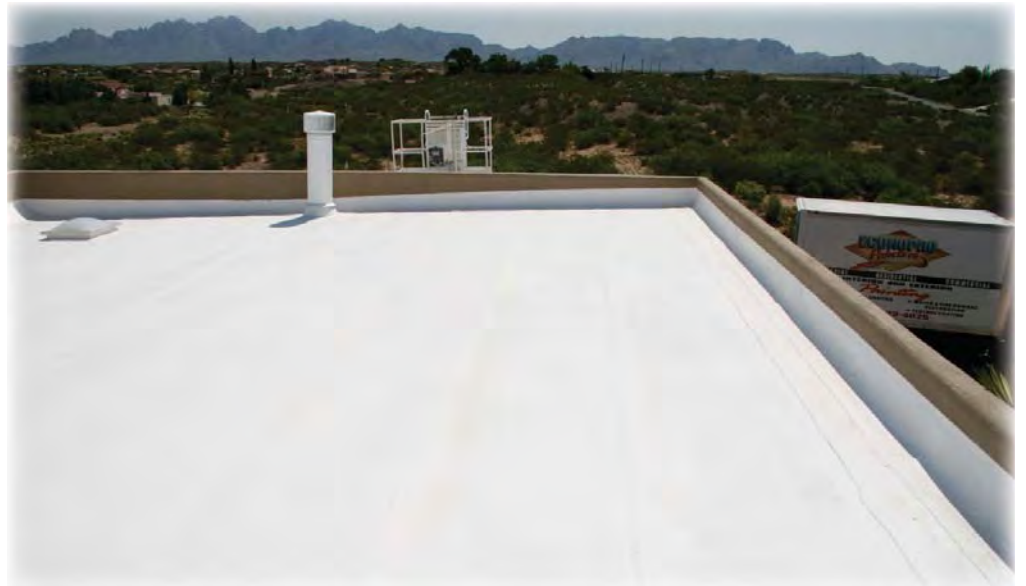
Before and after elastomeric roof coatings are applied on a commercial building in New Mexico. [Photos courtesy of Tim Waters, EconoPro Painters LLC]
