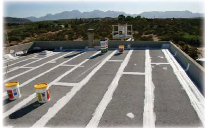
Before and after elastomeric roof coatings are applied on a commercial building in New Mexico. [Photos courtesy of Tim Waters, EconoPro Painters LLC]
