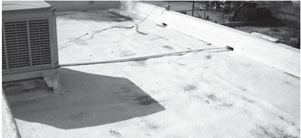
Note the contrast of dark areas and light areas and the foam domes, indicating a need to coat.
